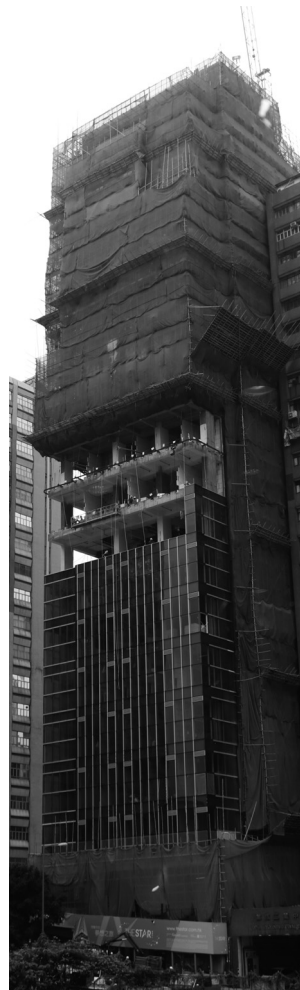
The Star under construction with topping out works completed
